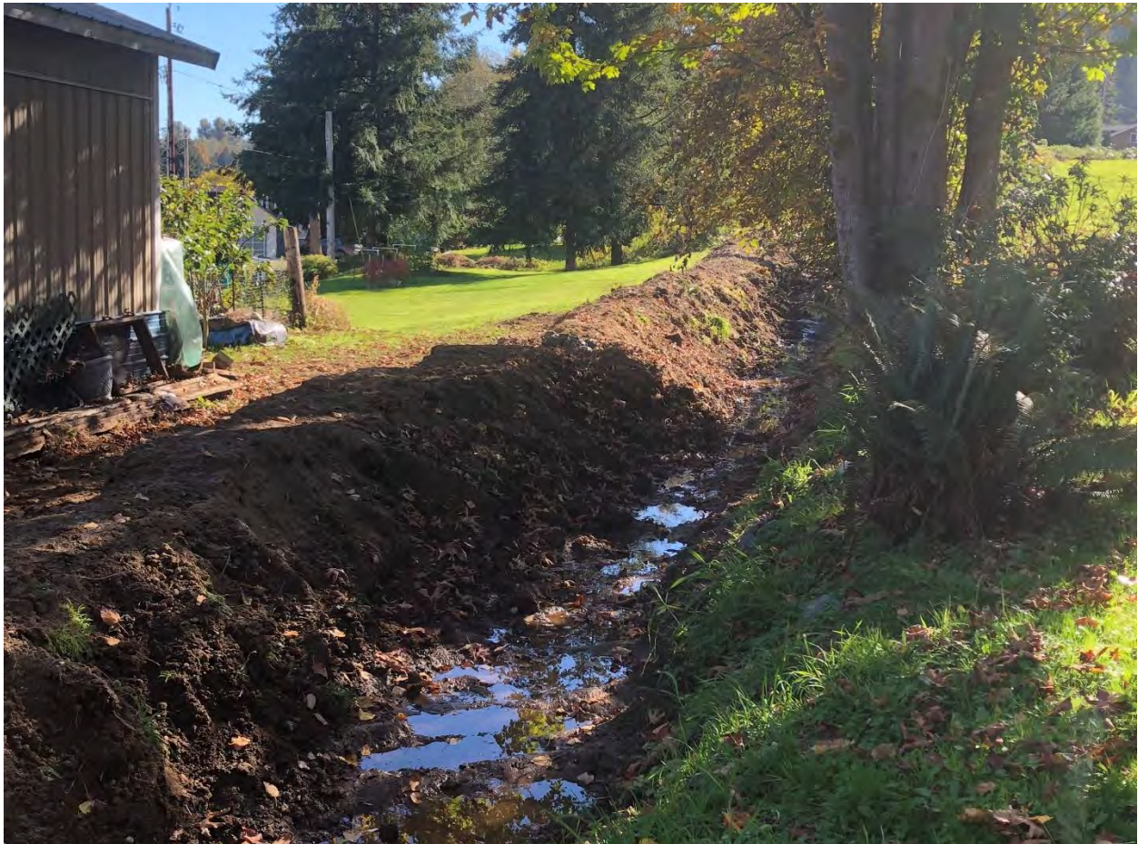
Photo 4. Unnamed tributary channel leading to Hull Drive shortly after it was dredged and the spoils placed to form a small berm along the east bank. (Photo provided by County, October 15, 2018).
