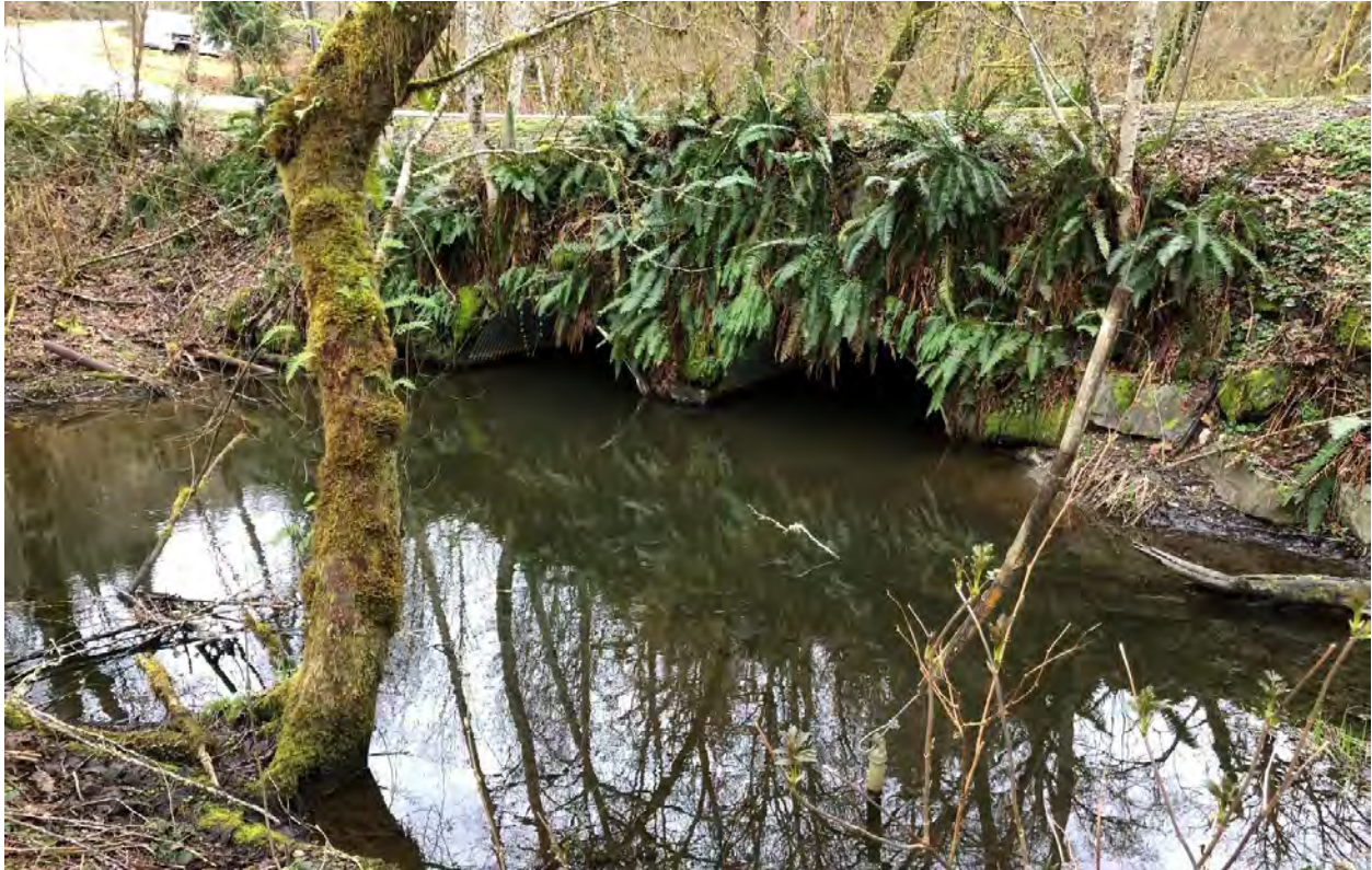
Photo 3. Outlet of existing dual culverts under McMurray Shore Drive.
