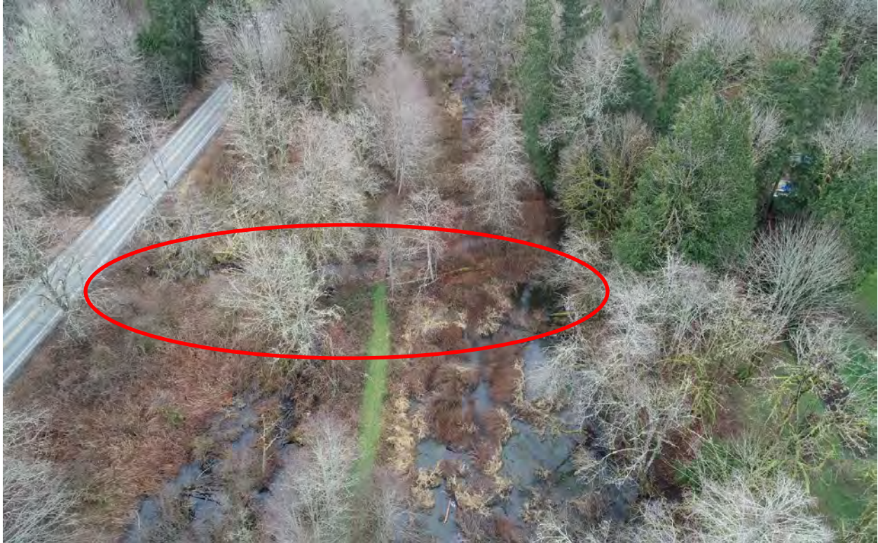
Photo 8. Looking downstream from McMurray Shore Drive. SR9 is on the left side of the photo. The green strip down the center of the photo is the top of the mainline abandoned railroad berm. The unnamed tributary is circled in red. (March 10, 2020).
