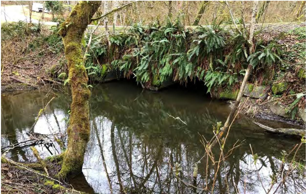
Photo 12. Outlet of existing dual culverts under McMurray Shore Drive.
